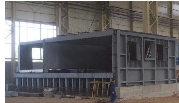
The shell of a 145 t dual-chamber melting furnace during installation
