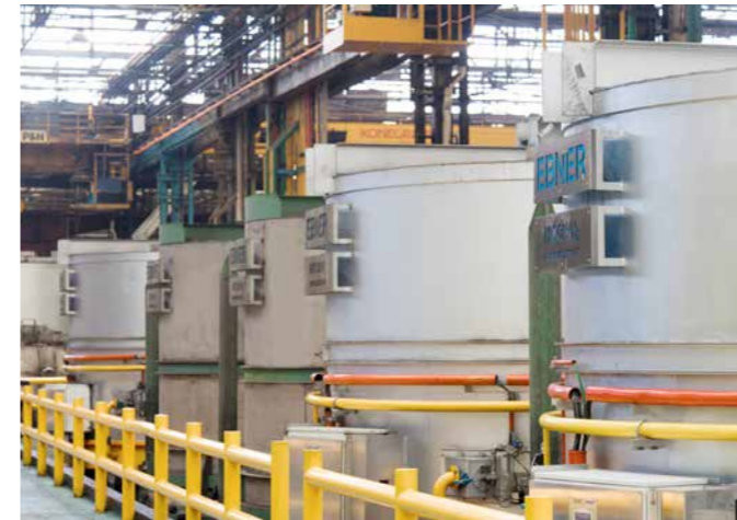
Nacobre trusts EBNER furnaces
